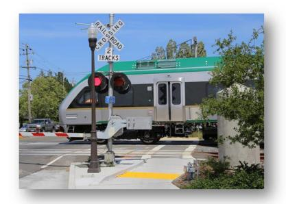
lights, gates and bells at each crossing. In total, more than 800 individual test train movements were made to demonstrate proper operation of the grade crossing warning systems.
