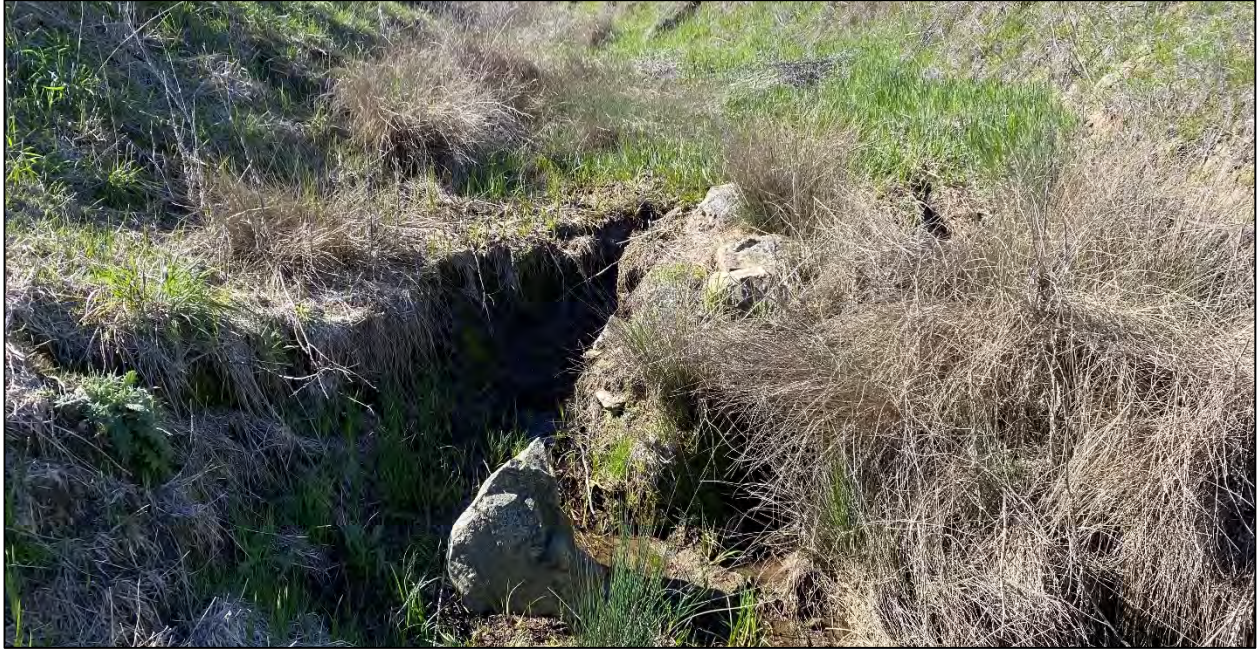
Photo 7: View of a headcut in the Windsor Drive Drainage. Photo taken on February 21, 2023.
