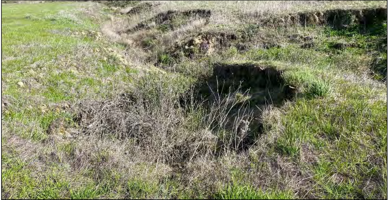
Photo 5: View facing northeast of bank failure in Windsor Drive Drainage. Photo taken on February 21, 2023.
