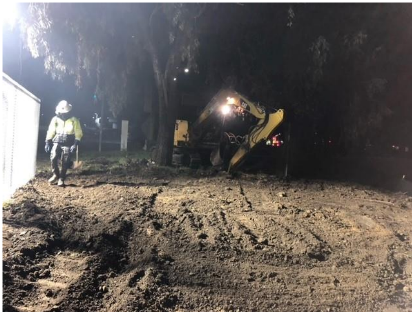
Site Excavating and Grading Ready for Planting along the San Rafael Creek
