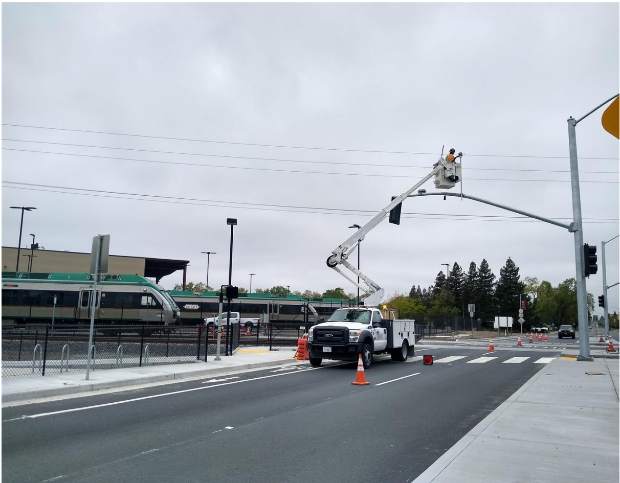
Traffic Signal Equipment Installation on Airport Blvd
