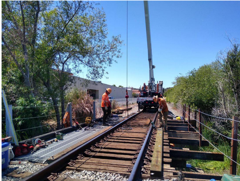
Replacing Timber Bridge Beams in Novato
