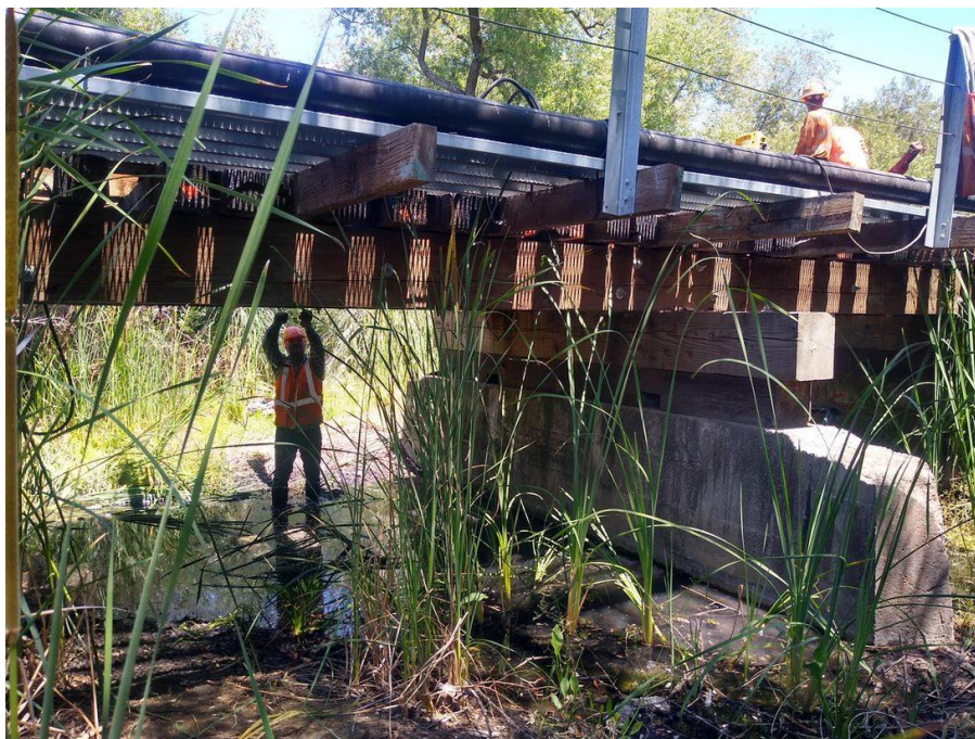
Bolting Down New Bridge Beams
