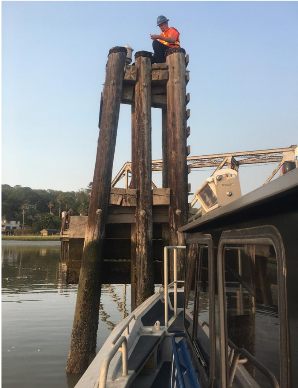
Blackpoint Bridge Fender Light Repair
