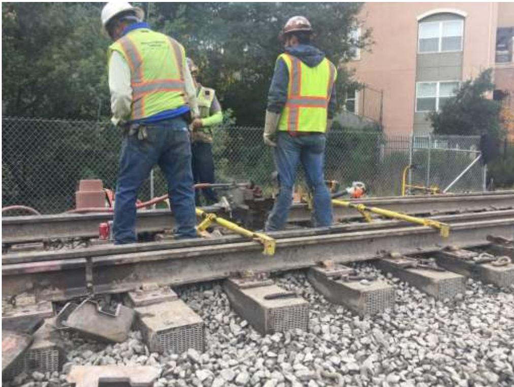
Track crews preparing to thermite weld gauntlet switches to existing rail.
