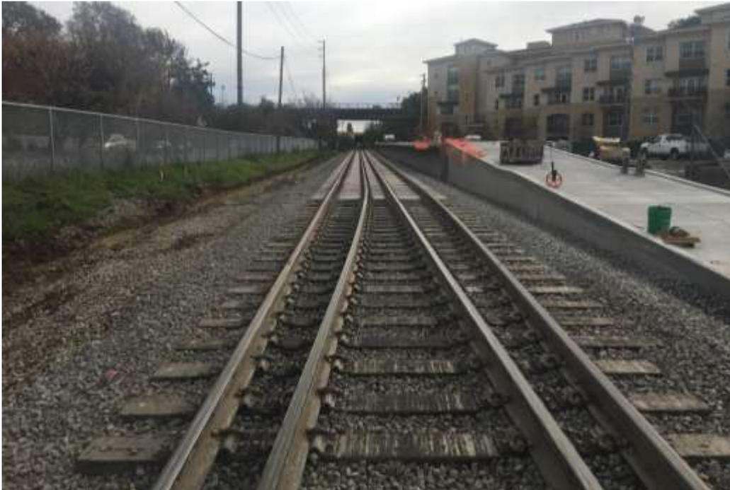
Track crews installed gauntlet switches and rail at north and south end of the station during weekend shutdown.
