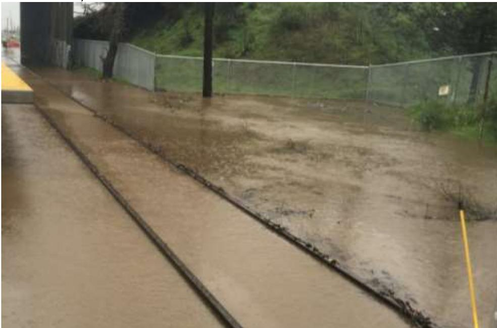
Flooding of the Civic Center Station trackway occurred when heavy rainfall coincided with a king high tide of the Gallinas Creek.
