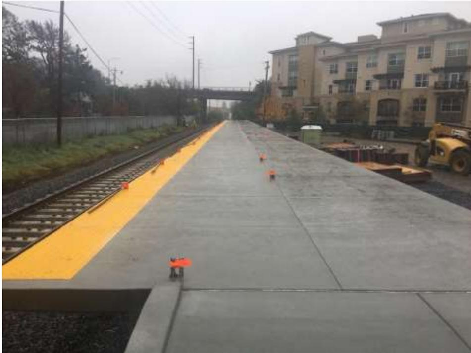
Completed concrete top slab pour and northern ramp.
