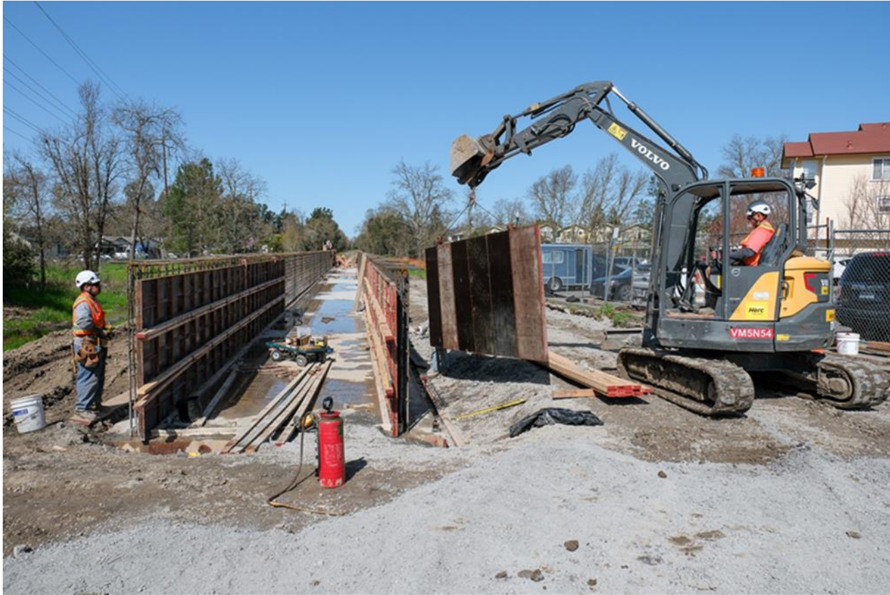
Setting concrete formwork for the Windsor Station platform
