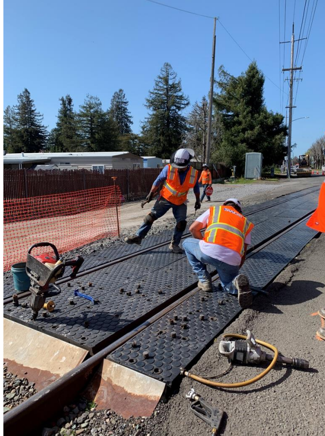
Removing bolts from the old crossing panels at McDowell Boulevard
