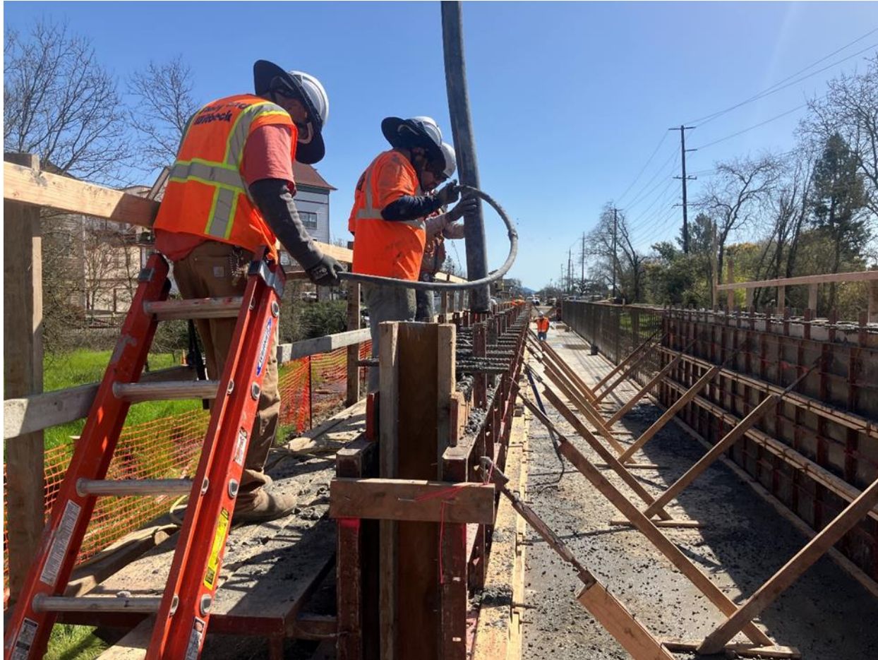
Placing concrete in the formwork for the Windsor Station platform
