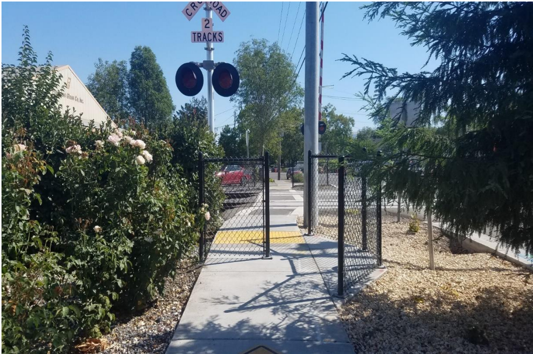
East Cotati Avenue, Cotati - Pedestrian Channelizing Fence
