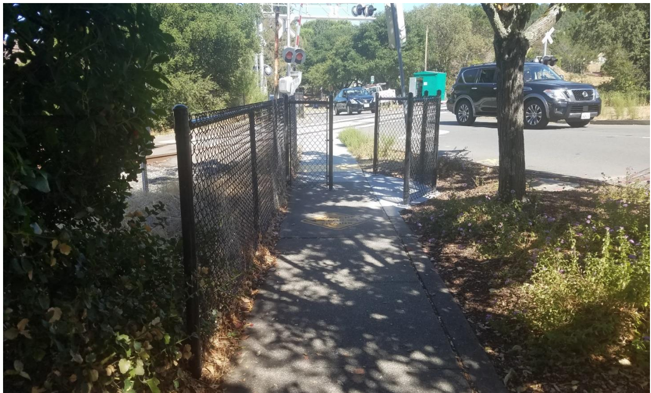
North San Pedro, San Rafael- Pedestrian Channelizing Fence
