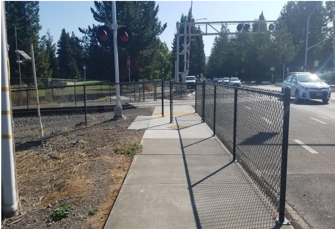
Rohnert Park Expressway, Rohnert Park- Pedestrian Channelizing Fence
