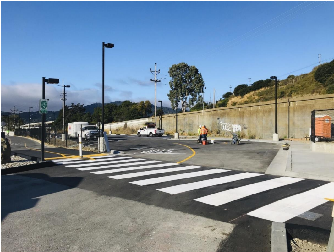
Larkspur Station Construction – Parking Lot Striping
