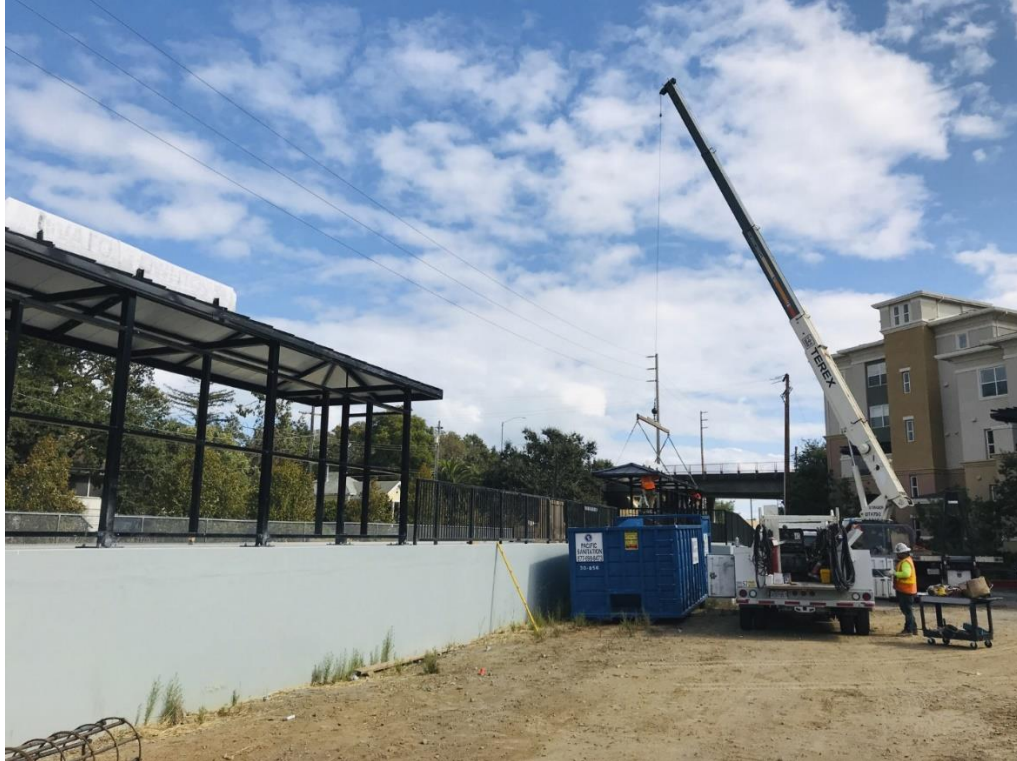
Novato Downtown Station- Shelter Installation
