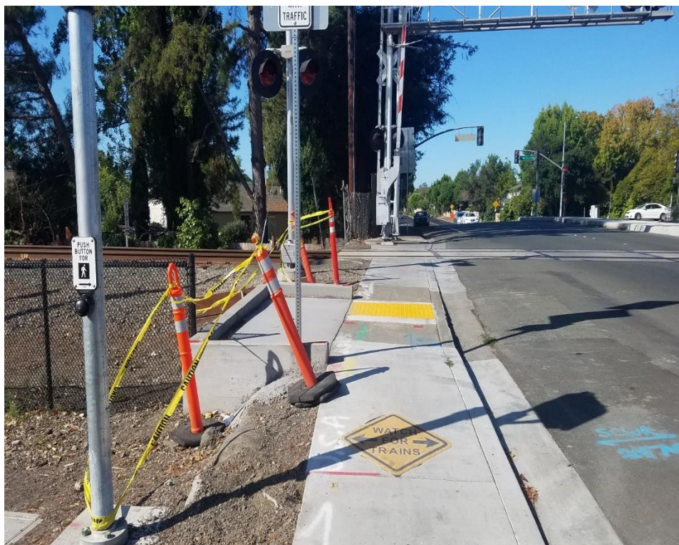
Southwest Blvd, Rohnert Park- Preparation for Installation of Pedestrian Channelizing Fence
