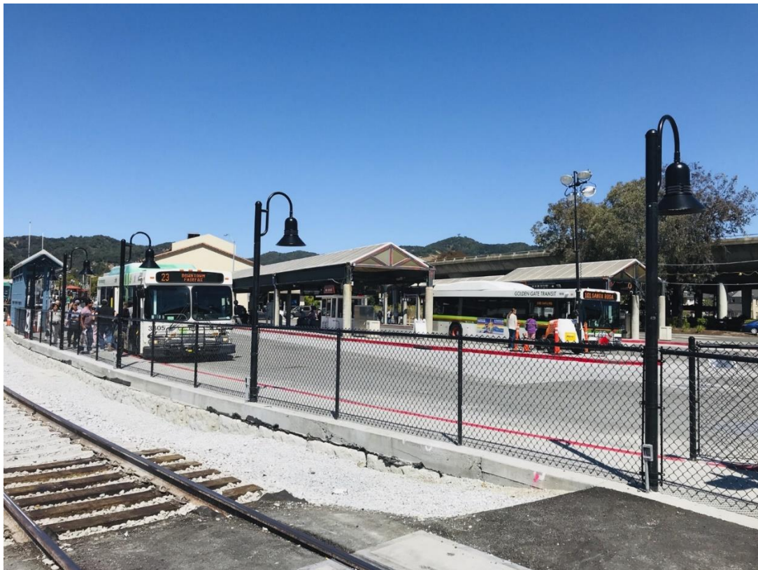
Bettini Transit Center – Lights Installed
