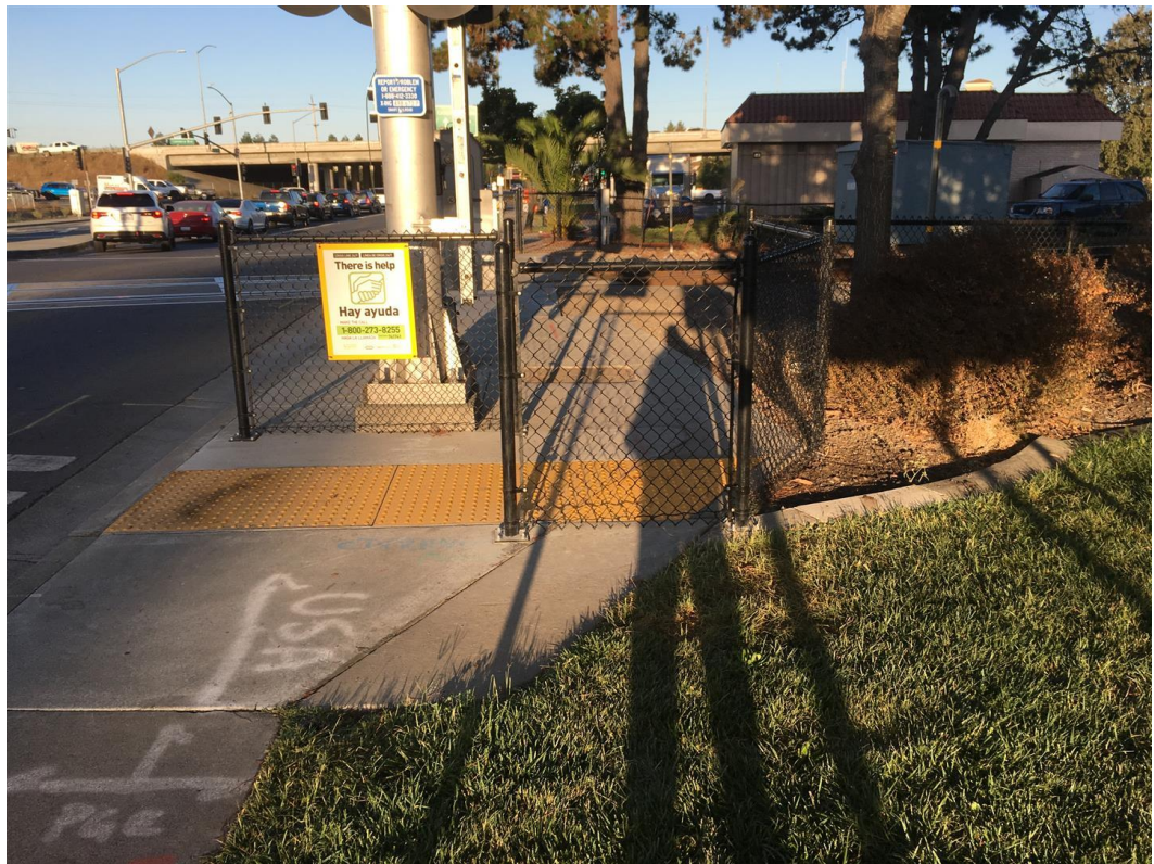
Golf Course, Rohnert Park - Pedestrian Channelizing Fence
