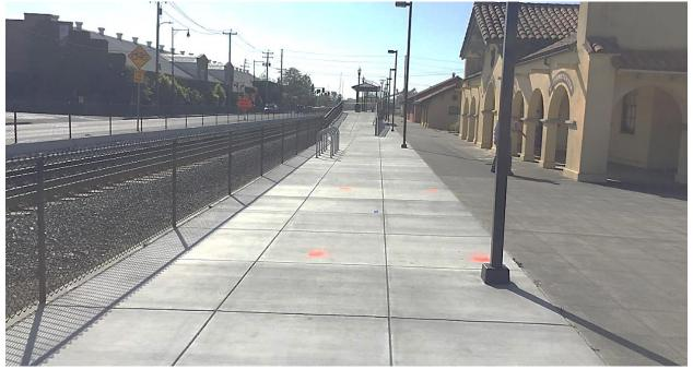
Orange paint on the concrete denotes the perimeter corners of where the electronic bike lockers will be installed.
