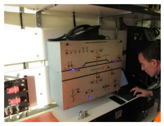
Signal Engineer verifying vital processor setup during testing, Santa Rosa
