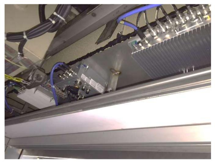
Installation of onboard Wi-Fi equipment
