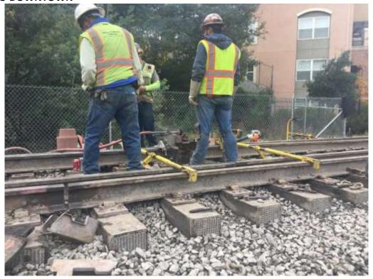
Track crews preparing to thermite weld gaunlet switches to existing rail.
