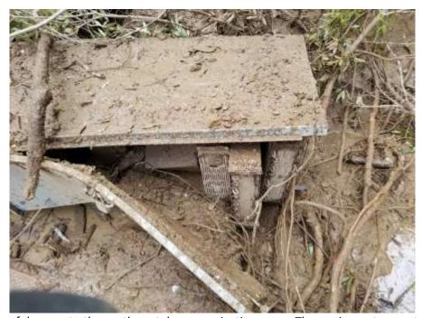
Close-up of damage to the north portal communications case. The equipment was a total loss.
