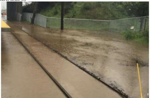
Flooding of the Civic Center Station trackway occurred when heavy rainfall coinsided with a king high tide of the Gallinas Creek.
