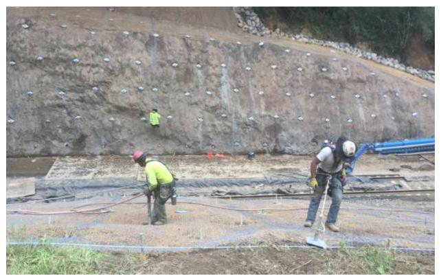
Crews are rappelling down the hillside to tighten the soil nail bolts in place.
