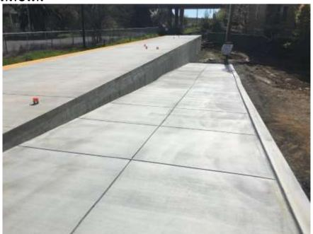
Concrete ramp pour completed at the southern end of the station.
