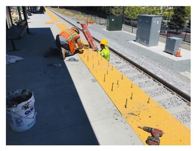
Larkspur Station Construction – platform edge warning tile installation
