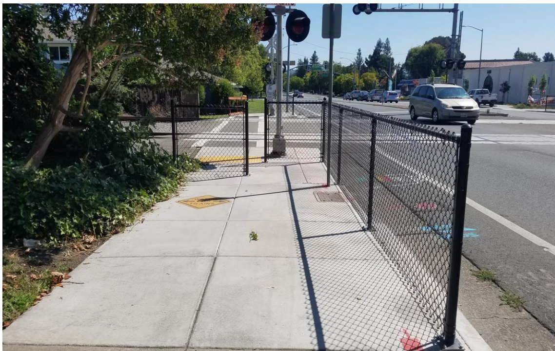
Guerneville Road Santa Rosa - Pedestrian Channelizing Fence
