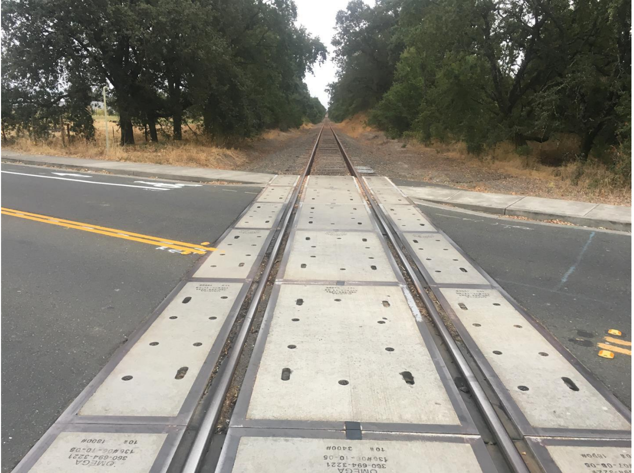
Windsor Extension - Mitchell Lane Grade Crossing current condition
