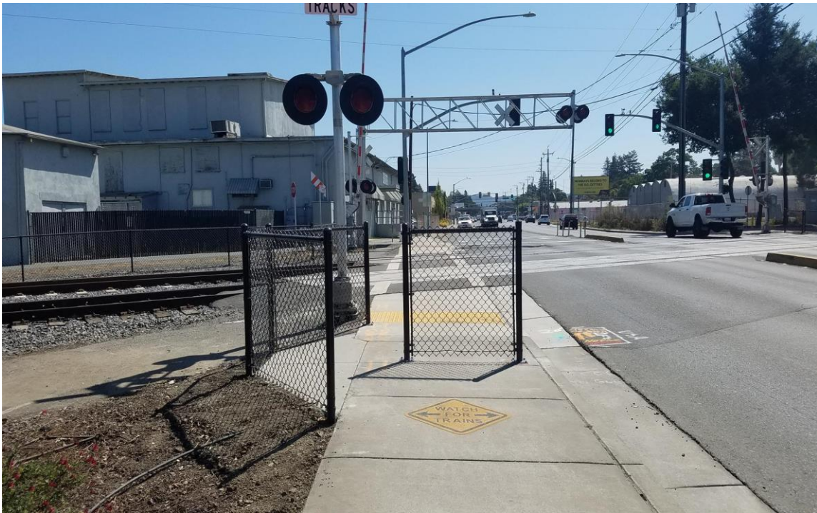
College Avenue Santa Rosa- Pedestrian channelizing fence
