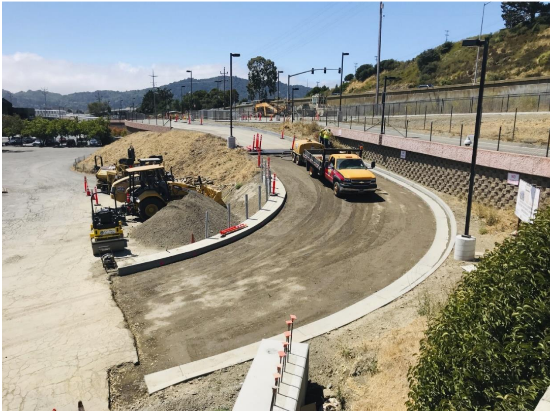
Larkspur Station Construction – Preparing for paving
