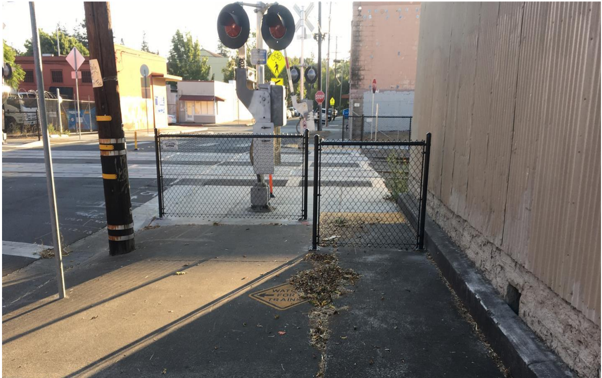
8 th Street, Santa Rosa – Pedestrian Channelizing Fence
