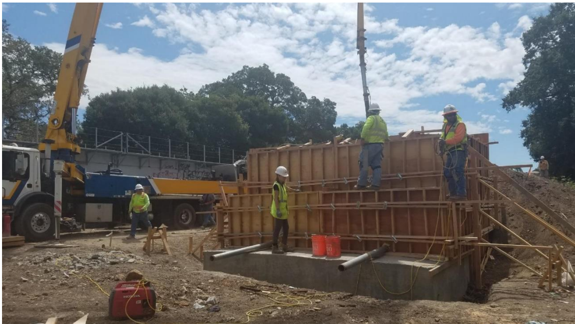
Pedestrian Bridge – North Abutment construction
