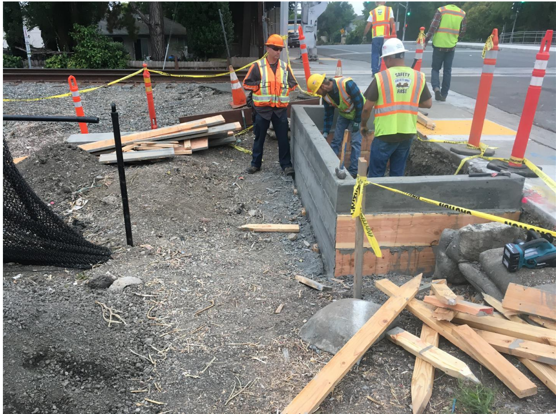
Southwest Blvd., Rohnert Park - Preparation for Installation of Pedestrian Channelizing Fence
