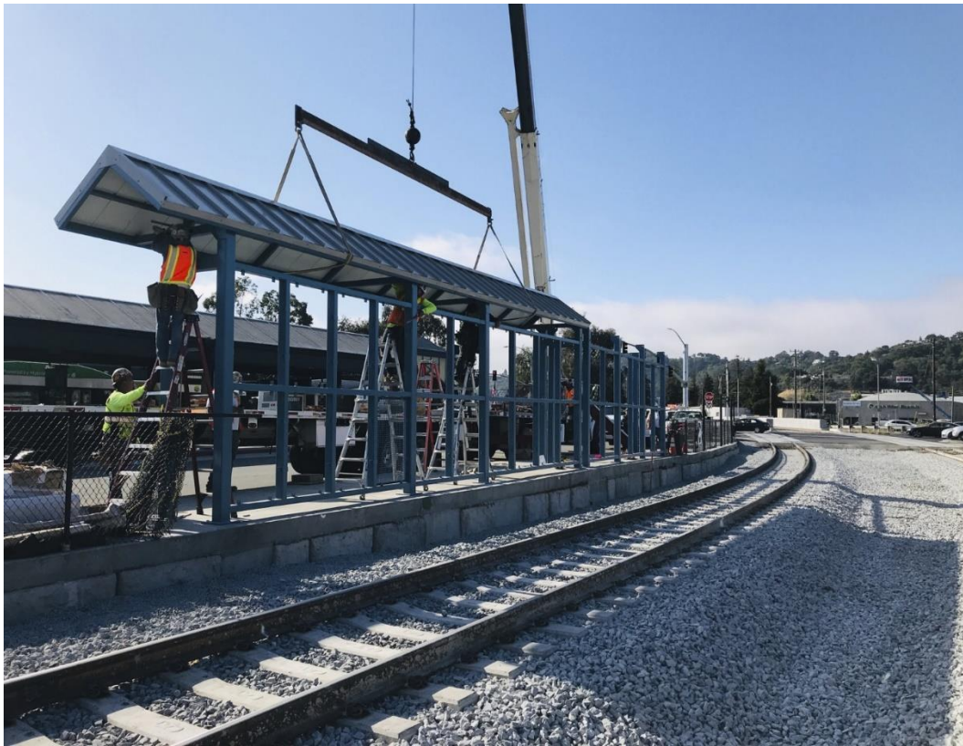
Bettini Transit Center – Installing a new Platform Shelter
