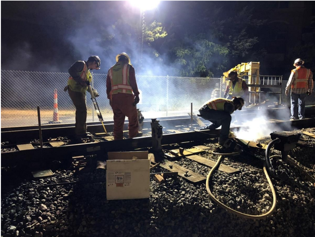
Novato Downtown Station - Track construction
