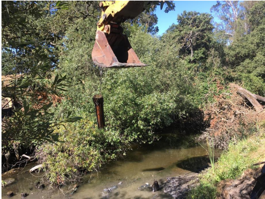
Old Pile Removal from the Petaluma River
