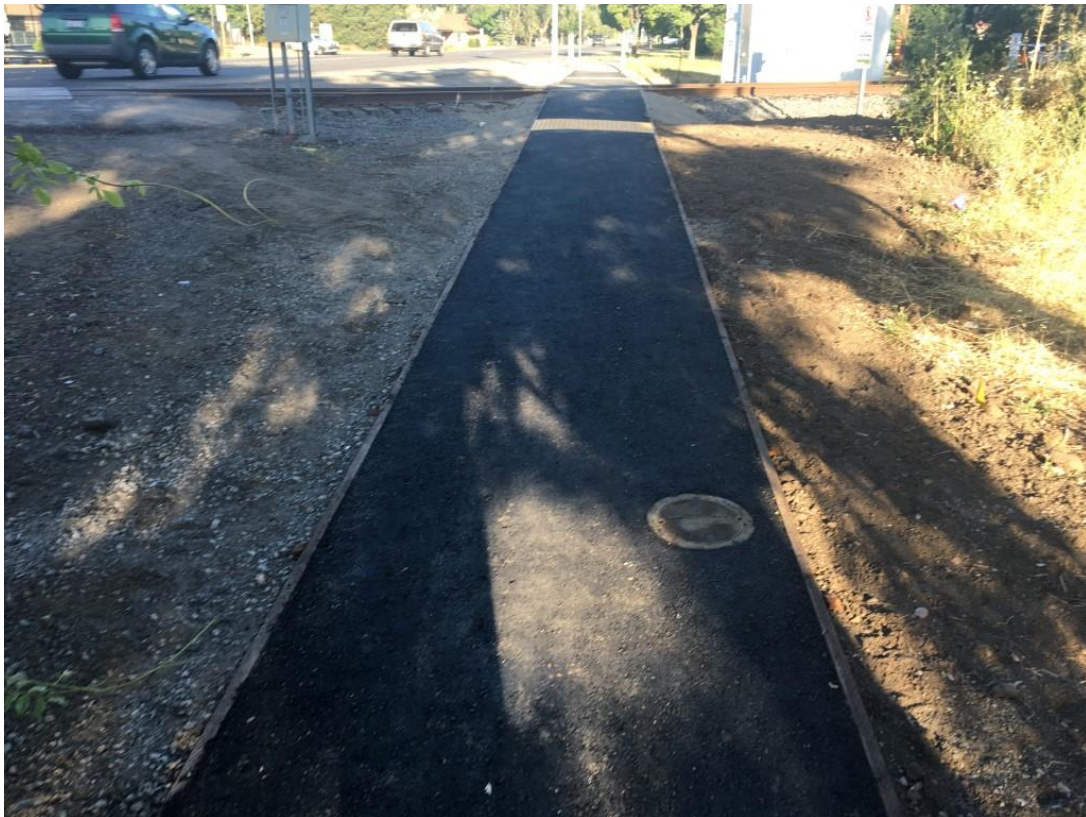
Construction of the sidewalk across the track on the north side of Airport Boulevard
