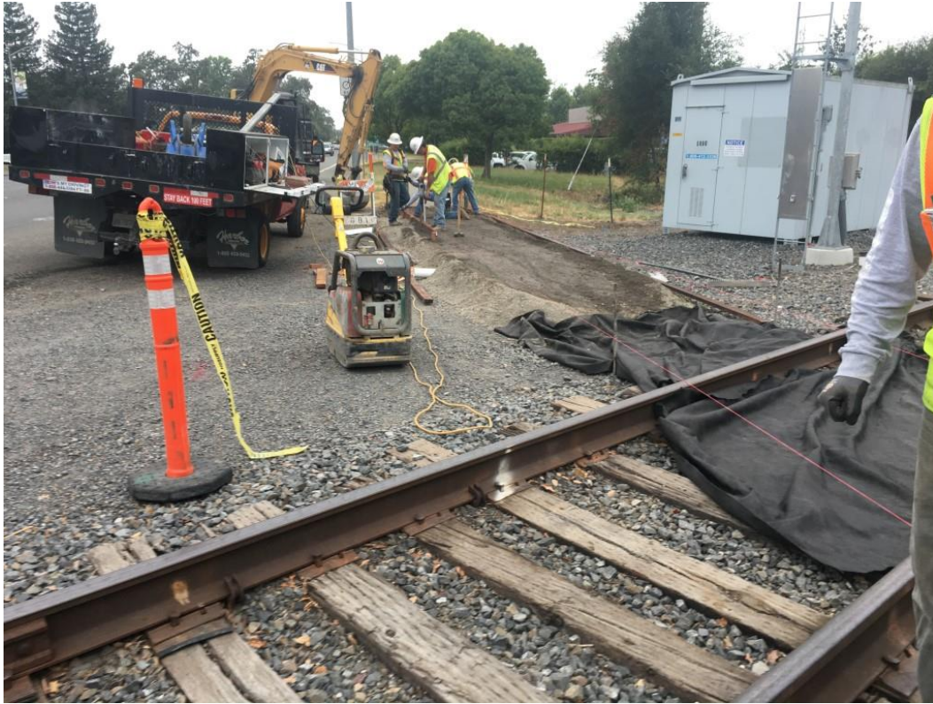
Construction of the sidewalk across the track on the side of Airport Boulevard
