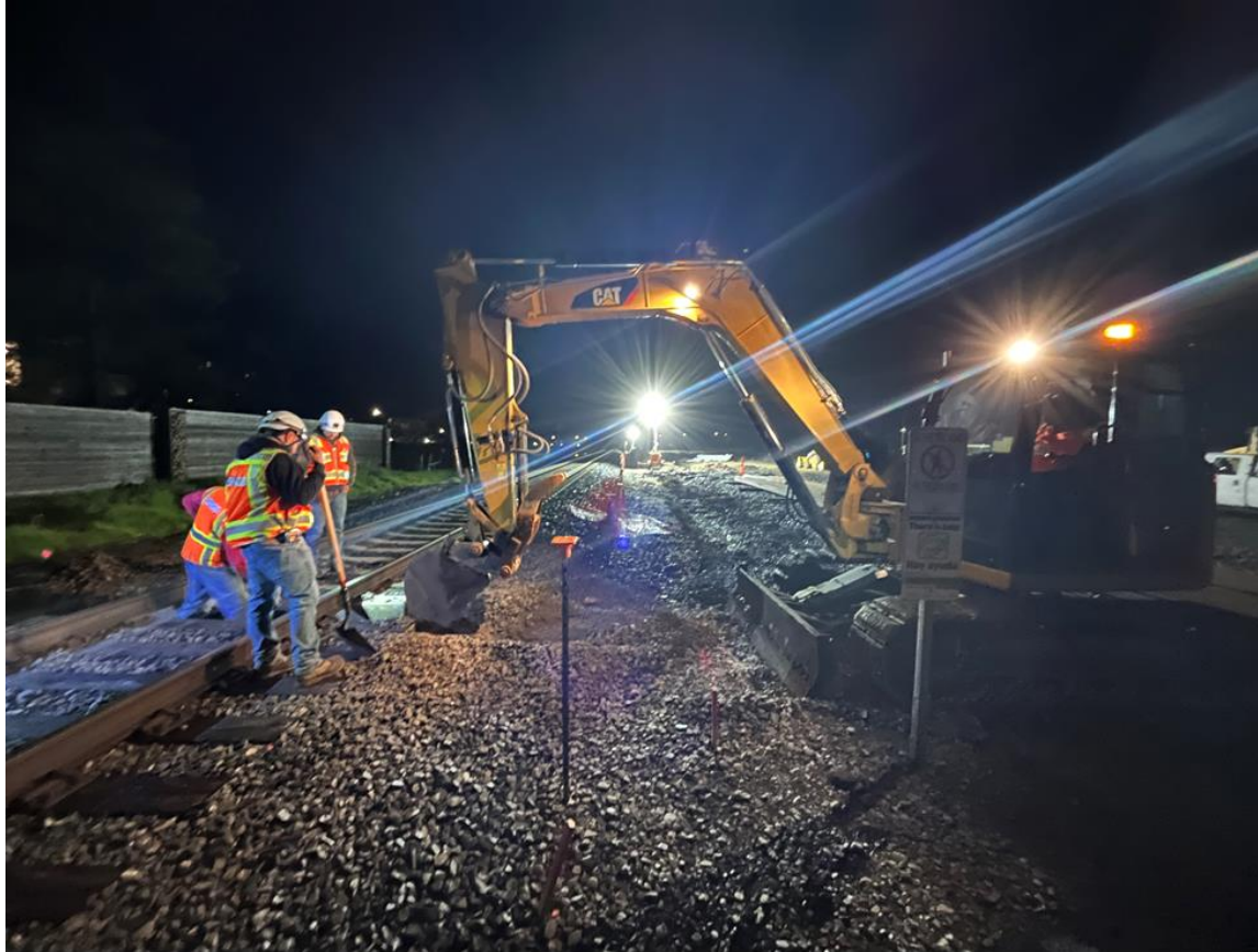
Contractor excavating underground conduit at Petaluma North
