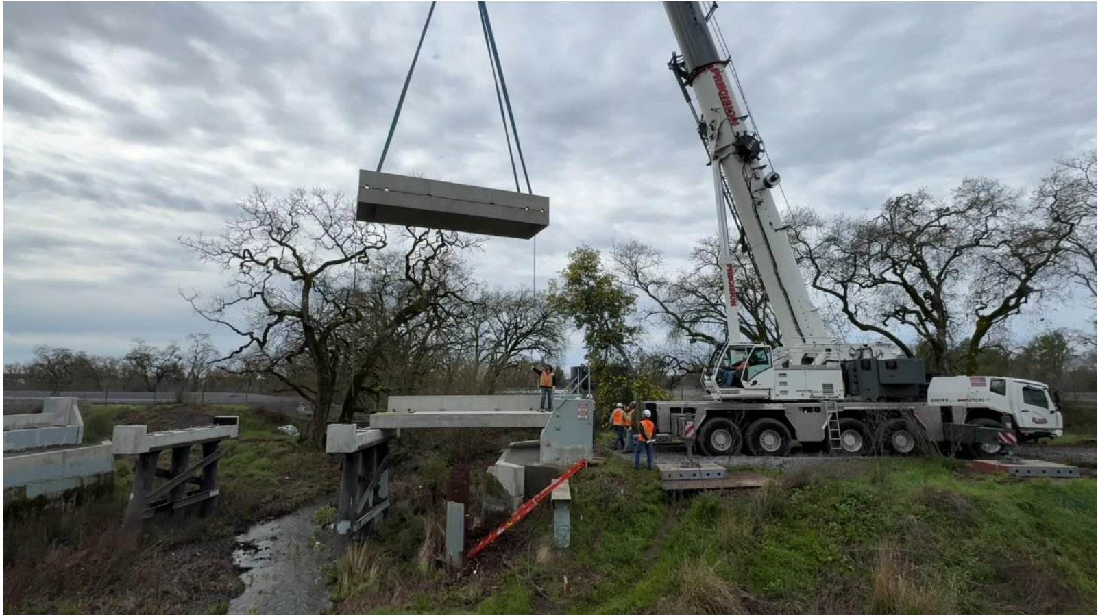
Setting bridge deck
