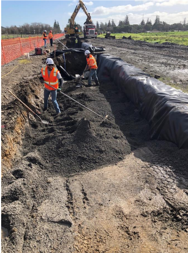
Excavation and soil/subgrade preparation for Petaluma North Platform foundation
