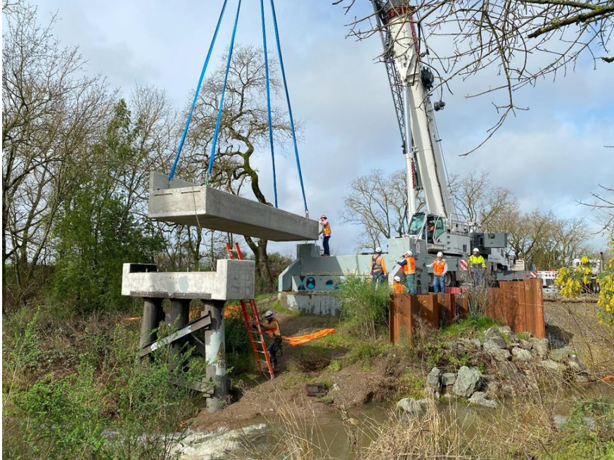
Setting bridge decks at Windsor Creek
