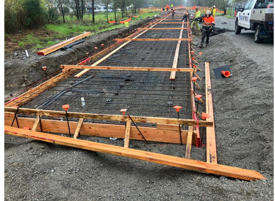
Concrete framework and rebar install for Windsor platform foundation
