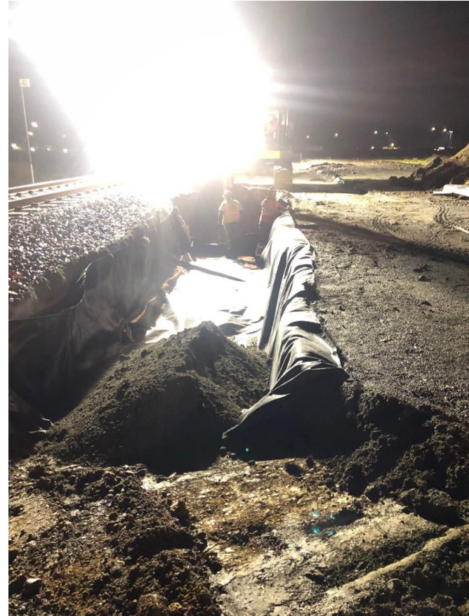
Excavation and soil/subgrade preparation for Petaluma North Platform foundation
