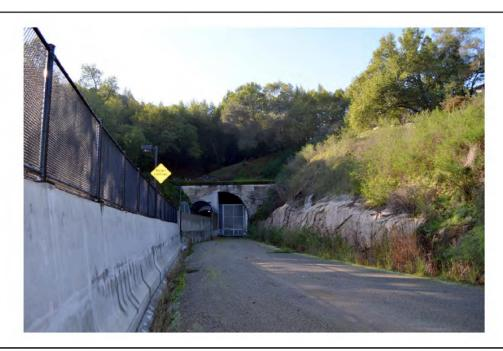
Photo 15: View of the alignment looking south at northern portal of the Cal Park Hill Tunnel. SMART ROW occupies the right side of the tunnel, the Cal Park Pathway occupies the left side.
