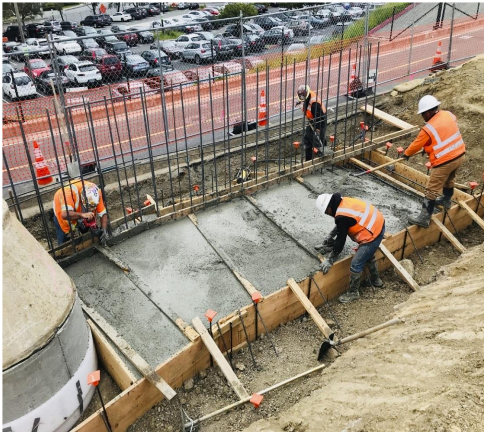
Retaining wall construction at the station site.
