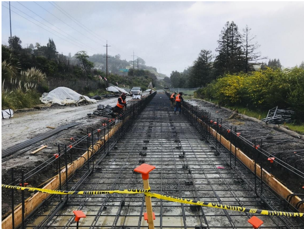
The Platform at the Larkspur Station is under construction.
