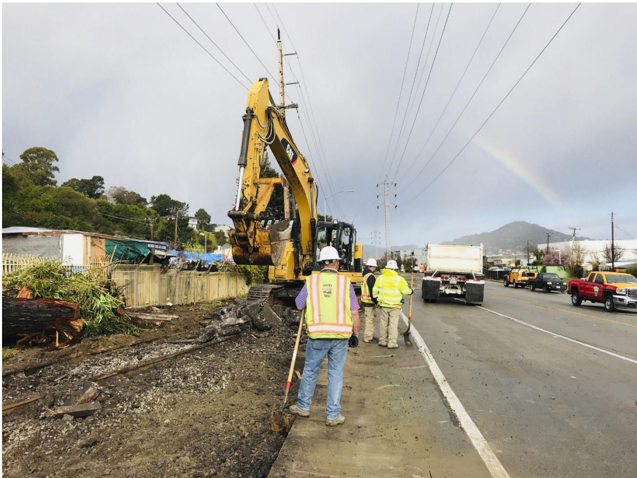
Andersen Drive Crossing Demolition
