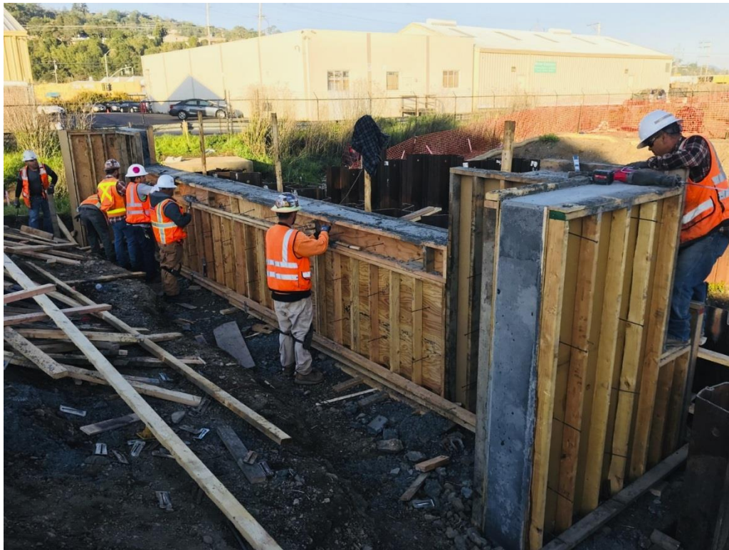
Unmaed Channel South Abutment is complete.
