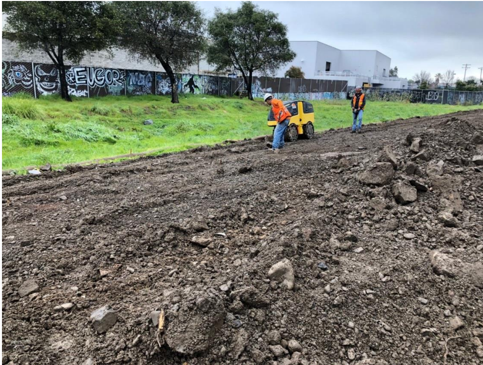
Unnamed Channel Bridge to Andersen Drive Ductbak Installation.
